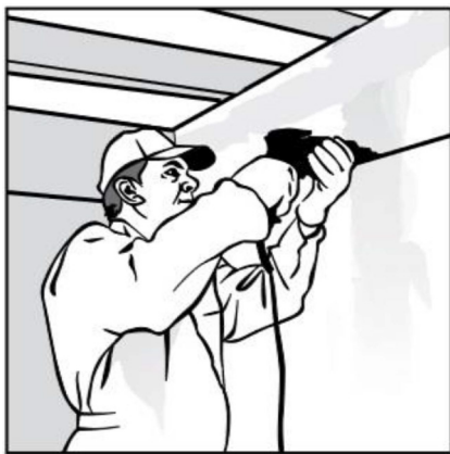
1. Fixing the perimeter L-channel
